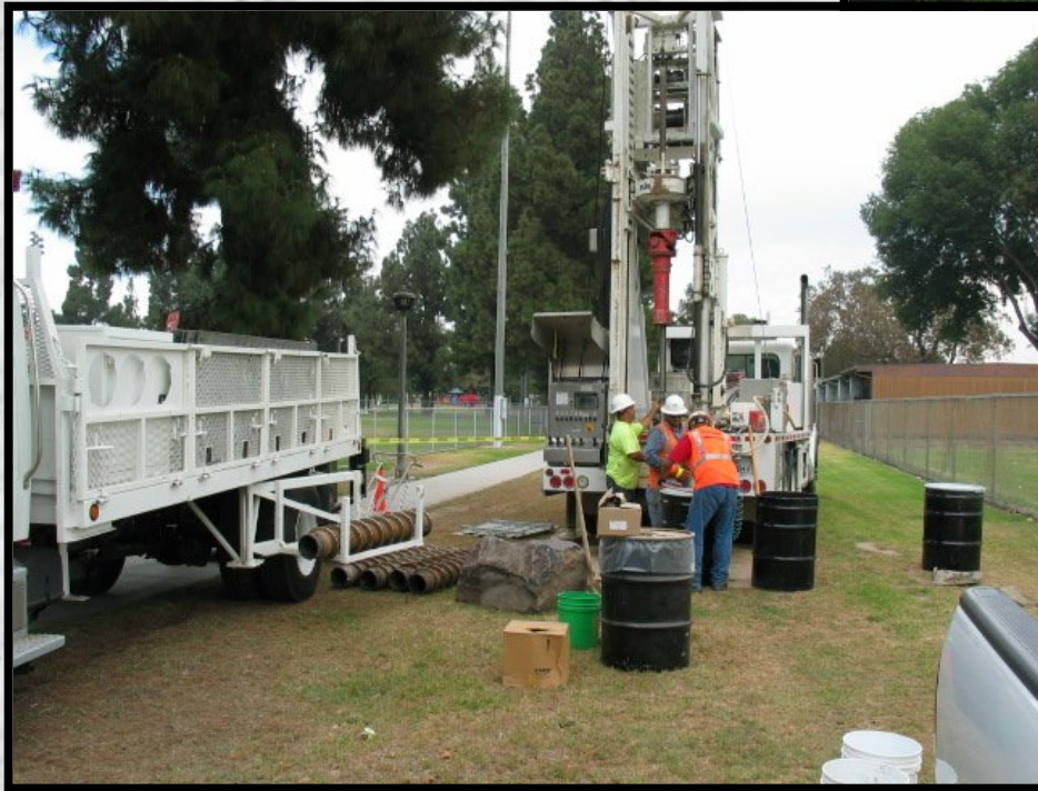
GMW-64 Hollow Stem Auger Drilling
